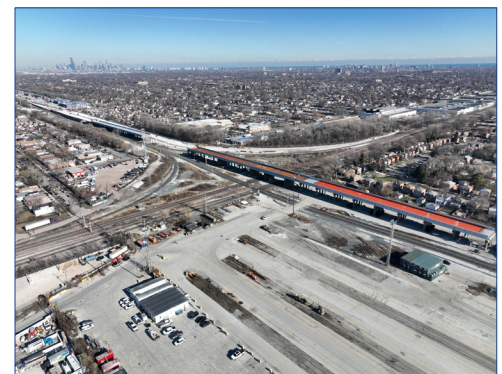
Forest Hill Flyover (P3) under construction.
